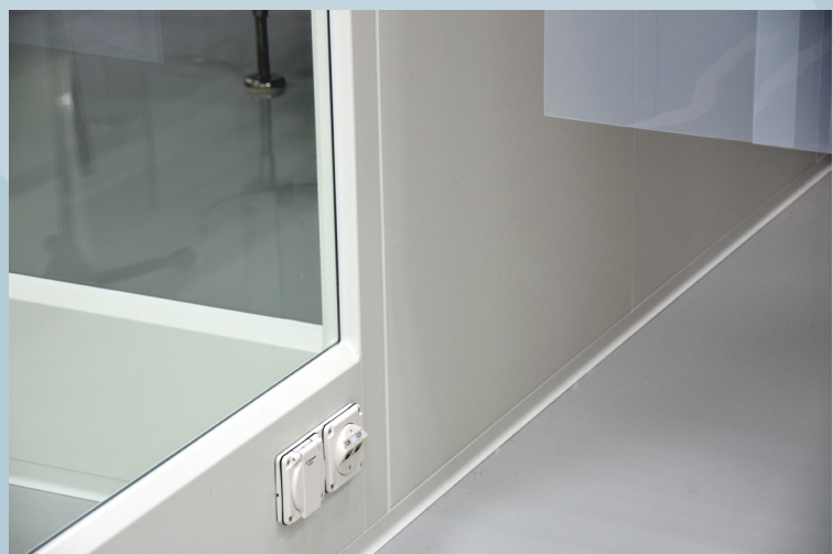
The interior is made out of materials such as glass, synthetic resin and stainless steel.
